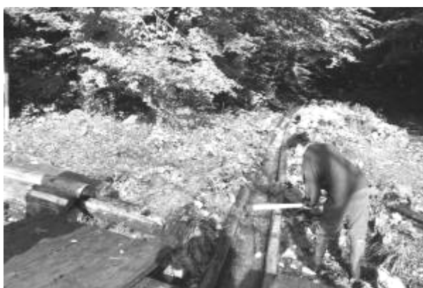
Fig. 6: Harmanec's water flume. There were used rods with metal hooks (sapina) for removing one metre logs from the water flume (photo by Jiří Junek)
