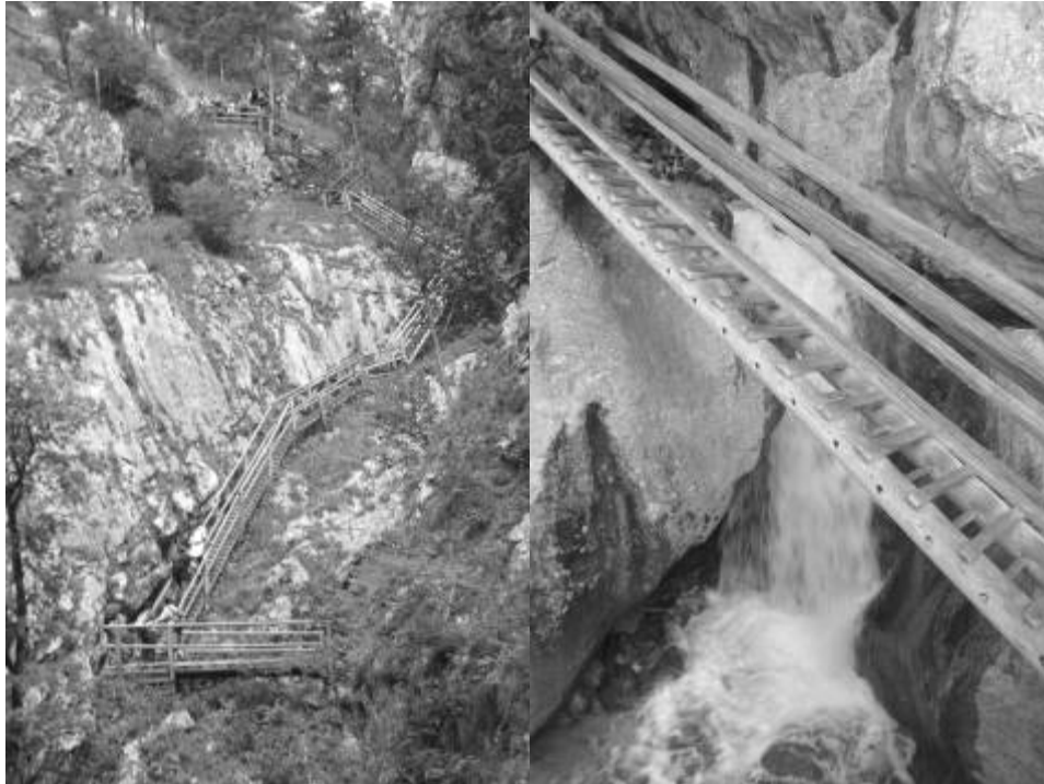
Fig. 4: Staircases and footbridges in the gorge
