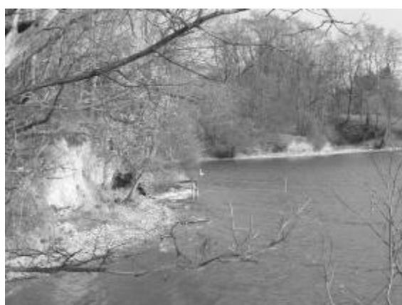
Fig. 1: Abrasion damaged bank of reservoir – limited of recreational uses (reservoir Brno, area Osada, foto M. Šlezinger 2012)
