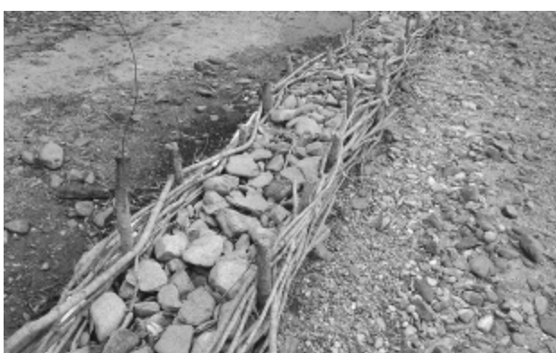
Fig. 2: Biotechnical stabilization - wattle work fence filled with stone – during construction in 2013 Photo M.Šlezingr
