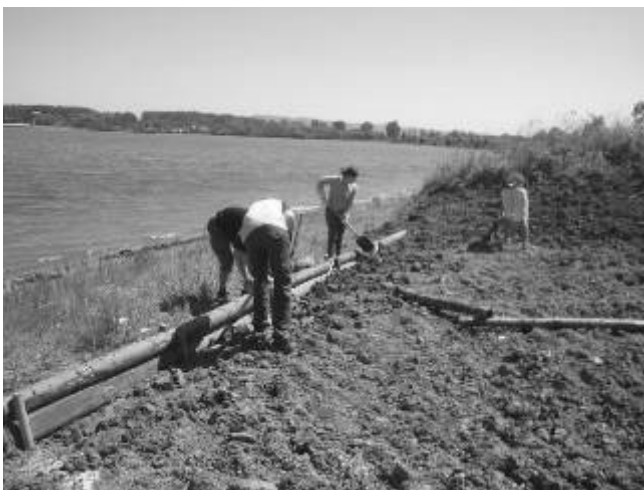
Fig. 1: Stabilization of bank, Hulín reservoir (gravel pit) (Photo M.Šležingr 2016, adjustments in 2017)
