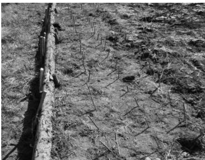
Fig. 2: Stabilization planting – Salix viminalis , 2 rows under stabilization, 3 rows above technical stabilization (Photo M.Šležingr 2017)
