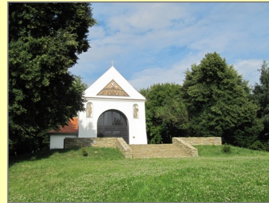
chapel sv. Rocha (after repair)
