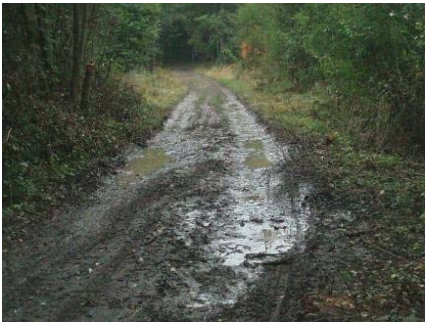
Fig. 1: The original condition of the forest road
