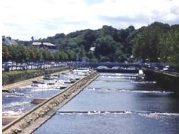
Fig. 3: Lannion whitewater stadium
