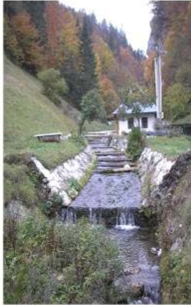
Fig.1 Sills in the torrent control Jelenec
