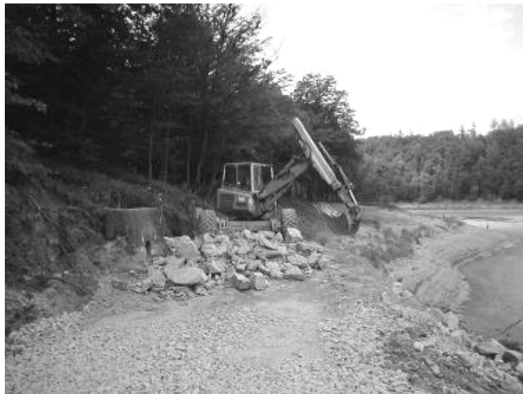
Fig. 3: Construction of bank stabilization while the Brno Reservoir is drained [11] [12]
